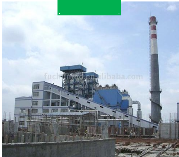
250 MW Power Plant
